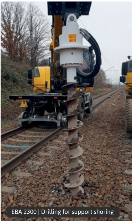
EBA 2300 | Special foundation work
