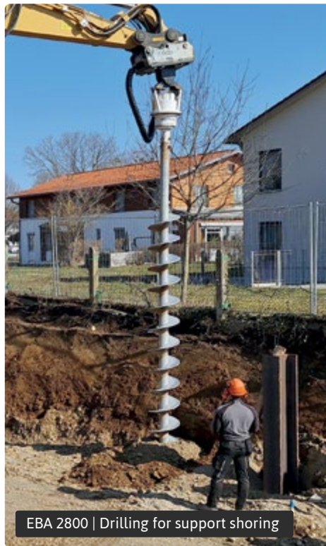
EBA 2300 | Drilling for support shoring
